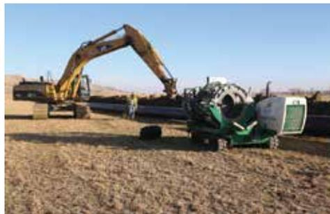
HDPE also eliminated the need for costly fittings and cut down on installation time due to narrower trench widths than those required for other piping materials.
